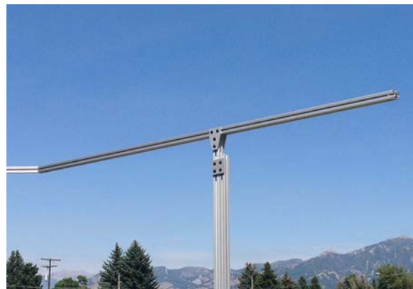
Figure 6: Custom-designed aluminum mounting strut frame top rail segments connected to expandable legs for 3 meter elevation.
