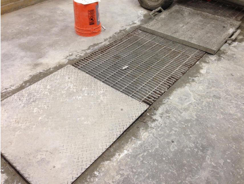
Fig. 7.5: Sump Inside Bulk Material Lab
